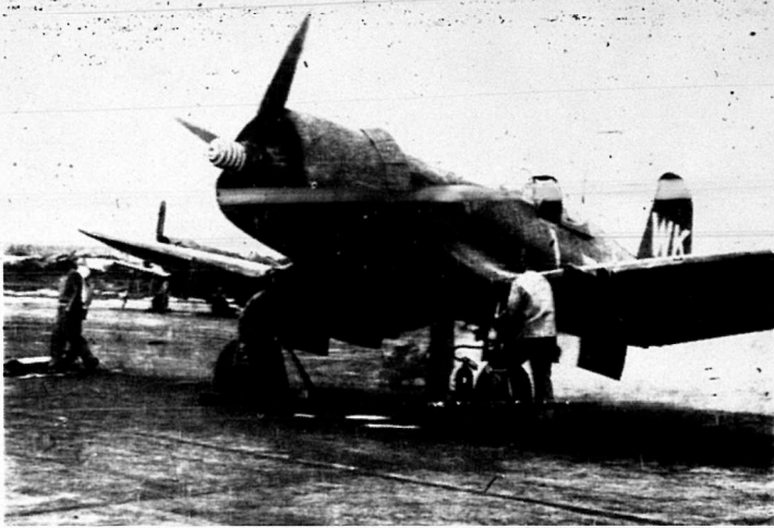
Undraft carburetion in the F4U-5 increases the danger of fire on starting, and therefore necessitates mechanics of Marine Fighter Squadron 224 working "in close" with their CO2 bottle, every-ready to extinguish any possible blaze at a moment's notice. TSgt. Eberle (facing camera), plane captain of WK-1 has just smothered a blaze and is set for another as the prop struts spinning through after a crank start.
