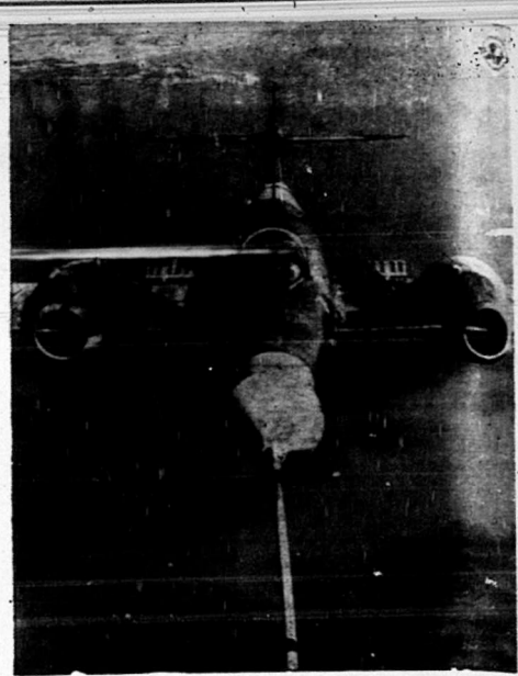
Refueled ten times in flight from a tanker plane this Meteor jet plane remained in the air for 12 hours and three minutes in southern England. Without refueling, the Meteor, Britain's fastest jet fighter, can stay in the air only 1 1/2 hours. Above, the nose of the jet is fitted by the pilot onto a metal cone fastened to the tanker, through which the fuel was pumped. This experiment was believed to have set a record for jet flight endurance.
