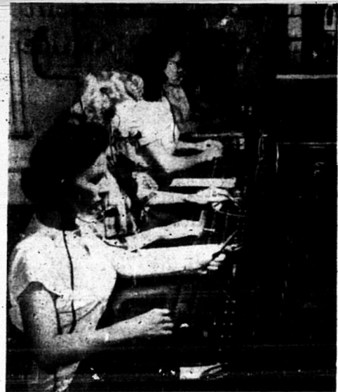
"Number please!" query these efficient telephone operators who keep the lines humming at Cherry Point. (Left to Right) Edna Kilborn, Margaret Yates, Betty Lamb and Wilma Chelf. The switchboard which handles incoming and outgoing calls for more than 1350 phones here on the station is one of the most up-to-date boards in this part of the country. —(Photo by SSGT "Gus" Dazentials)
