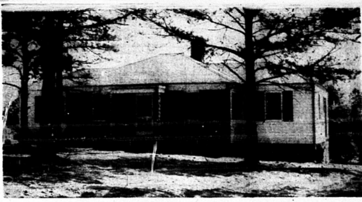
The above house is one of the several various styled dwellings which are now being constructed in the Havelock Housing Project. Manufactured by the Knox Corporation of Thomson, Georgia, the semi-prefabricated structures have been approved by the Federal Housing Authority throughout several states. They are constructed from wood having a moisture content not greater than 19 per cent and are completely insulated.
