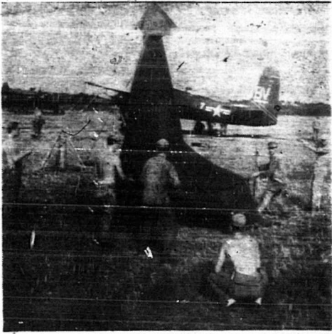
—Staff Photo SETTIN' UP CAMP will be the order of the day soon when 2nd Wing heads south for fleet exercises. Photo shows erection of VMP-354 "line shack" at Roosevelt Roads last year.
