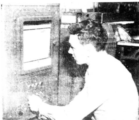
Looking over the new cellometer gear, an electronic device for measuring cloud ceiling, is PFC James C. Davis of AFS-16. The 25,000-watt candle-power beam is projected from a bulb smaller than a cigarette and may also be used as a night navigational aid.
