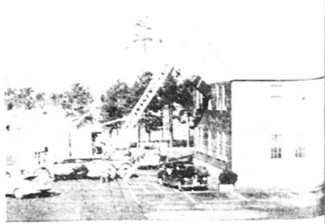
Workers are shown lifting by crane a safe to place in the recesses of 601 and 602 of the 2nd Marine Aircraft Wing in the Aviation Administration Building. The picture was taken from the office of the Windsock.
