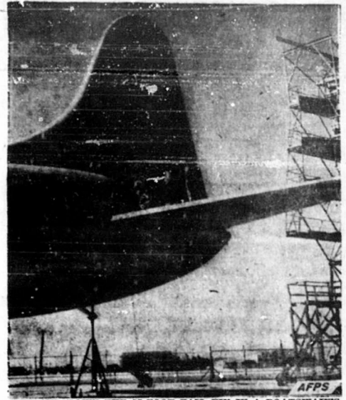
UP AND DOWN THE 57-FOOT TAIL FIN IN A BOATSWAIN'S CHAIR WILL BE PART OF STANDARD MAINTENANCE PROCEDURE ON THE AIR FORCE'S NEW XC-99. THIS 133-TON, 6-ENGINE SKY GIANT, CAPABLE OF HAULING 400 SOLDIERS OR 1000,000 POUNDS OF CARGO, IS ARE WORLD'S LARGEST LAND PLANE. IT IS BEING FLIGHT TESTED AT THE PRESENT TIME, AND WILL SOON BECOME A PART OF THE AIR FORCE FLEET IF IT COMES UP TO EXPECTATIONS.
