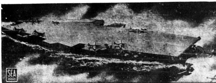
THE NAVY'S NEW 65,000 TON CARRIER will look somewhat like this artist's conception when completed. Minor deviations may be made from the above drawing but at present the Navy's plans correspond with this interpretation. The ship has been awarded hull number CVA 58. It will be the largest U. S. naval vessel ever constructed and will be 130 feet longer on the waterline than the 45,000-ton Midway-class carriers.
