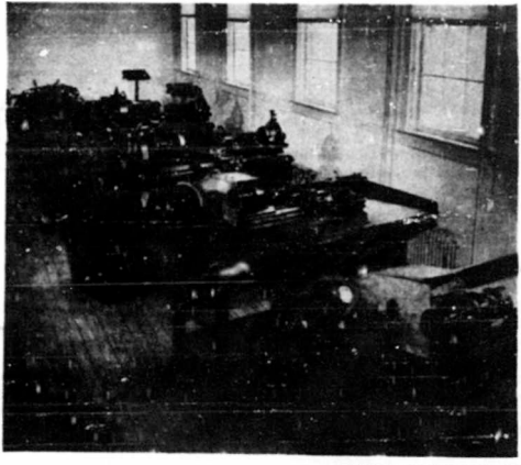
—Photo by Dagenais, PIO Some of the power equipment in the machine shop section of the Hobby Shop located in Bks. 227 directly behind the Ad Building Parking lot (former WR area).
