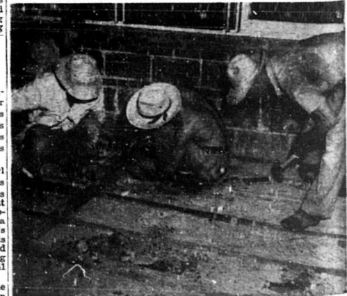
WORKMEN of civil service Public Works work laying down the floor of the new Officer's Club now under construction. They do one of the many tasks handled by civilians here.
