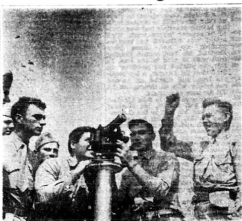
UPPER AIR SOUNDINGS are made by students of the Aerology class recently organized in the Operations building. Taking the view through the theodolite is Pvt. Jack Keller, while Pvt. Frank Zsoldos prepares to release the helium balloon.
