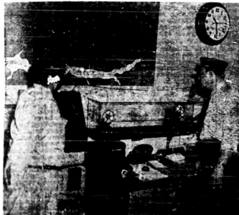
ALARM BOARD situated in the Fire Chief's office indicates the locale of a reported fire instantly and directs the rolling trucks to the scene of action with no time wasted.
