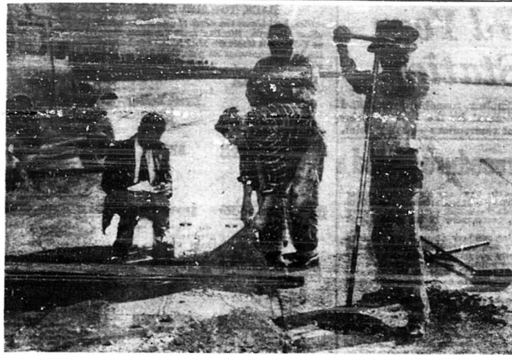
CIVILIAN workers attached to operating unit two of the Airfield Evaluation Program sink a shaft through one of the station's air strips to obtain a "soil profile," or cross section, of the underlying earth.
