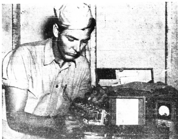
Radios must be checked thoroughly after each flight. Loose connections could cause a crash landing and loss of a plane. Corp. Back runs tests on this apparatus.
