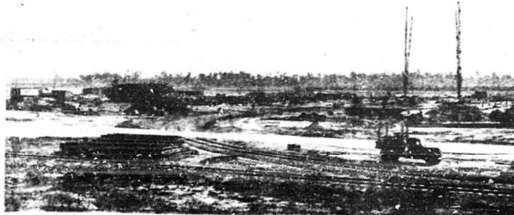
Barren and littered, this was the site of the A & R buildings when construction of the huge project began.
