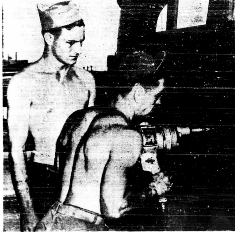
DRILL HOLES in the new sheet metal siding and upright of a bus are bored by Sgt. Alfred Santilli, NCO in charge of the body shop. Pfc. Cullen F. Gentry assists.
