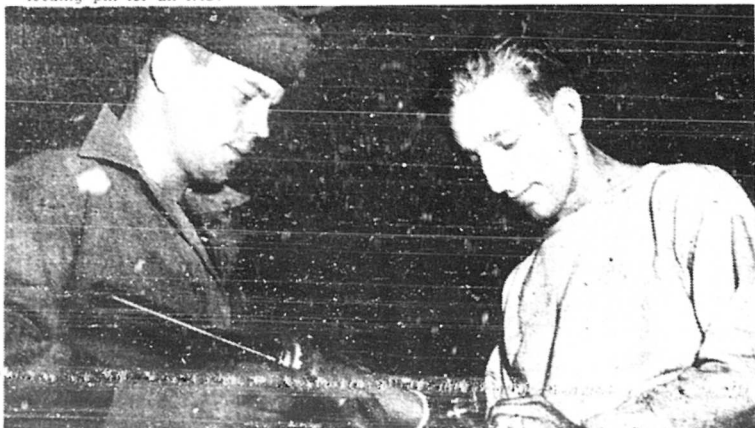
Sgt. George Lewis and Pfc. Nicholas Ricciardi work on an actuating cylinder for an SNJ in the Hydraulics shop. Here are checked and repaired all hydraulics equipment in the various planes, mainly for flap control and landing gear.
