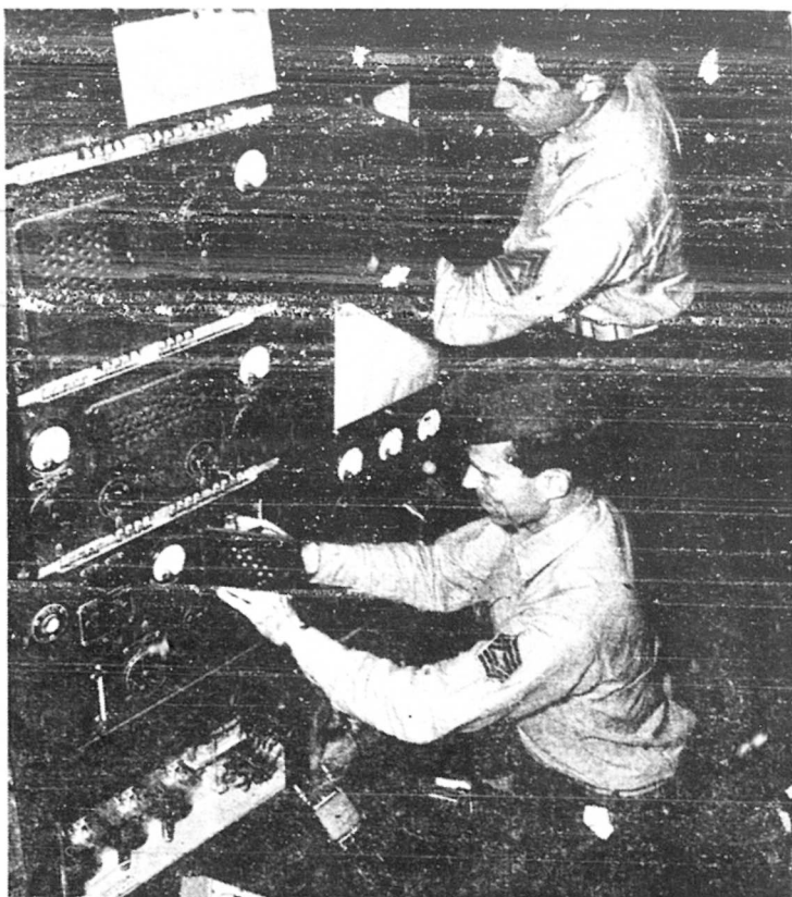
Finishing touches on the installation of 1,000-watt transmitter prior to applying voltage are given by MT-Sgt. Mortimer S. Sumberg and T-Sgt. Irwin Solomon
